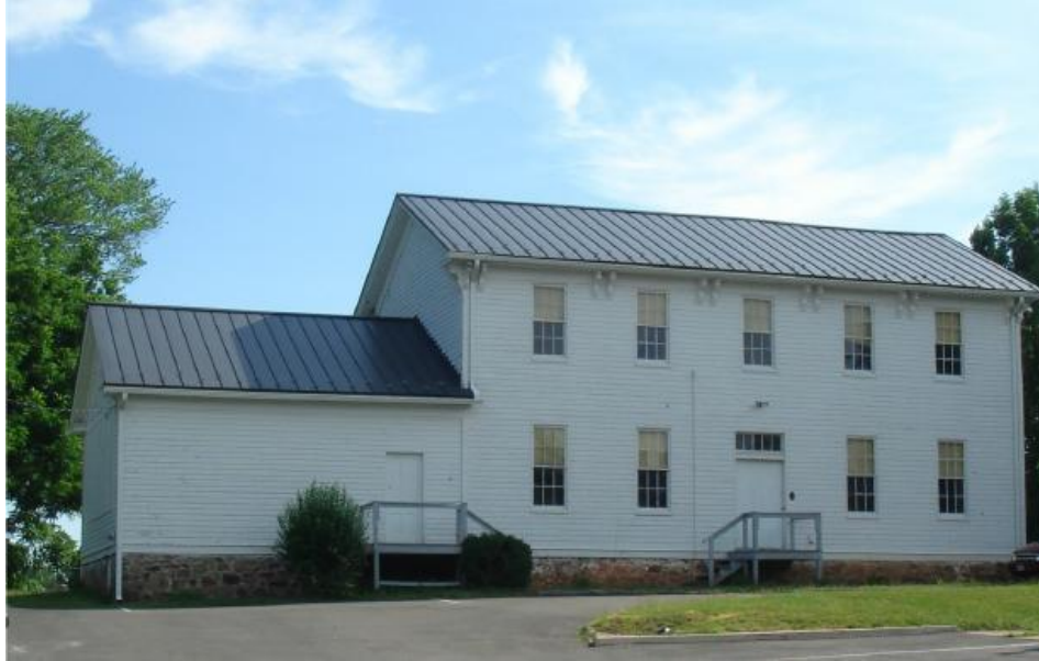
Figure 3 Union Street Building - Now used for storage
